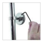
Screw the 5" or 8" shower head to the shower head arm taking care not to damage the plated surfaces. Carefully tighten the shower head with a suitable spanner or a tool with smooth jaws just sufficiently to lock the head in position.
